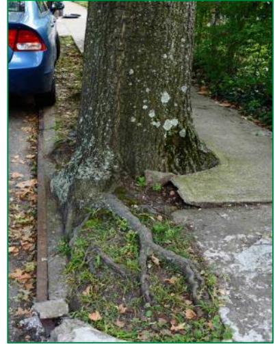
Photograph 16. Large tree species planted in small spaces, such as this pin oak, can lead to sidewalk damage.
